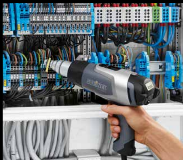
Shrinking cable sleeves in distribution cabinet
