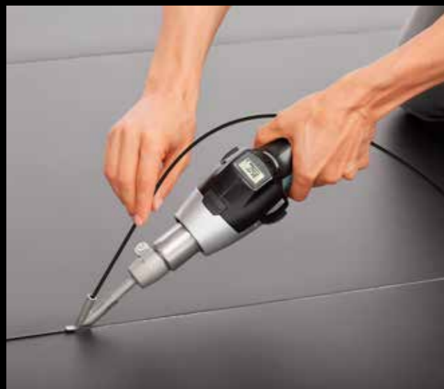
Welding linoleum floors.
