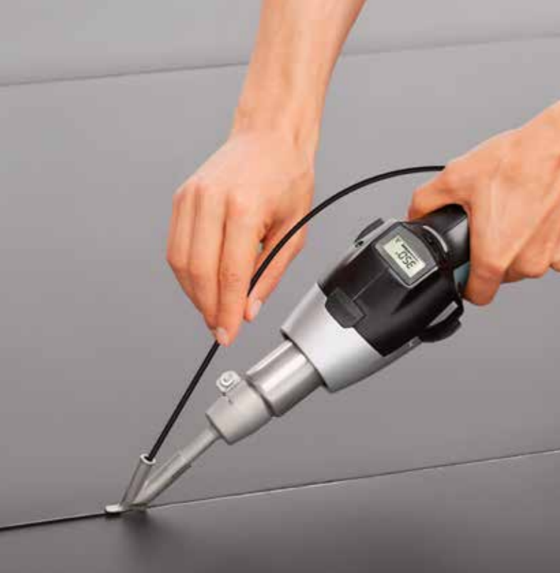
▲ Welding linoleum HG 2620 E
