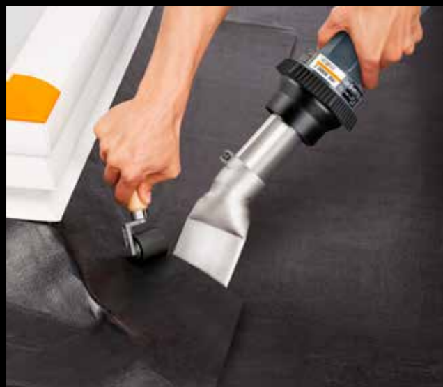
Overlap welding on a light dome.
