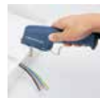
Cutting out small cable channels
